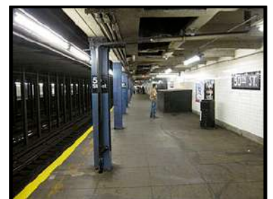
Platform Intrusion Detection
