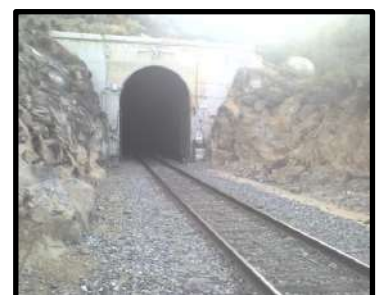
Tunnel Intrusion Detection
