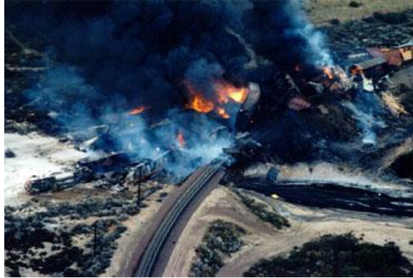
Rail cars carrying hazardous material exploded on bridge
