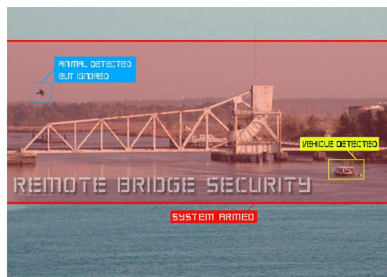
Remote Bridge Monitoring and Control
