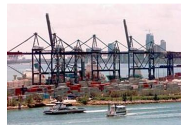
Seaport with HAZMAT terminal facilities
